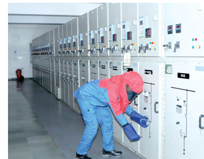
Use of Arc Suit during EHV Operations
