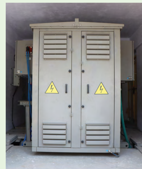
Dry Type Distribution Transformer to reduce mineral oil utilization
