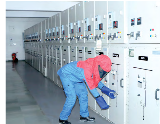
Use of Arc Suit during EHV Operations
