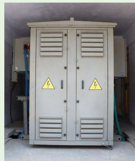
Dry Type Distribution Transformer to reduce mineral oil utilization
