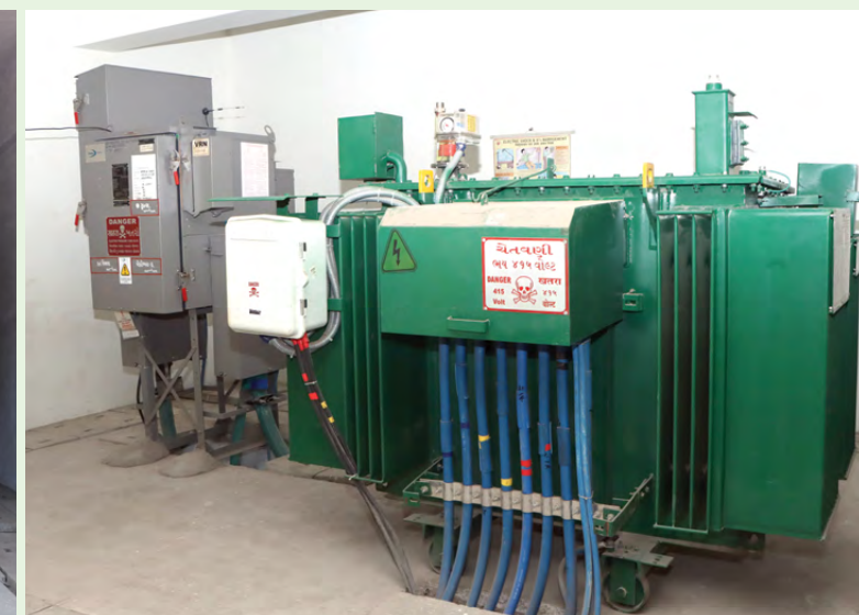
Environment-friendly Hermetically sealed Natural Ester oil filled Distribution Transformer
